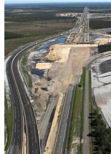
Autoroute A63, France
