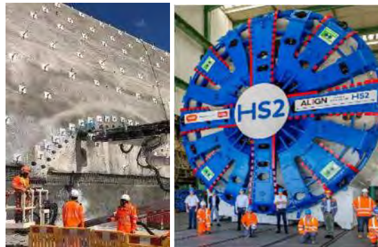
Section C1 – HS2 high speed railway line – United Kingdom (€1.1bn) b
