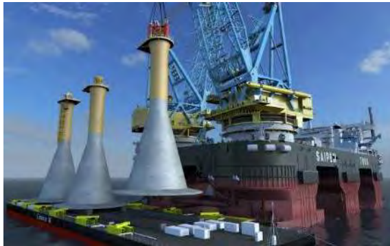
Design, construction and installation of 71 foundations for the future offshore wind farm at Fécamp – France (€552m) a
