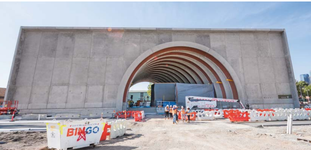
← In early 2022, fifteen arches made of 104,000 locally manufactured bricks were erected at the entrance to Arden Station, in northern Melbourne.
