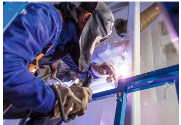
↑ An employee of an Equans partner company welds supports.
