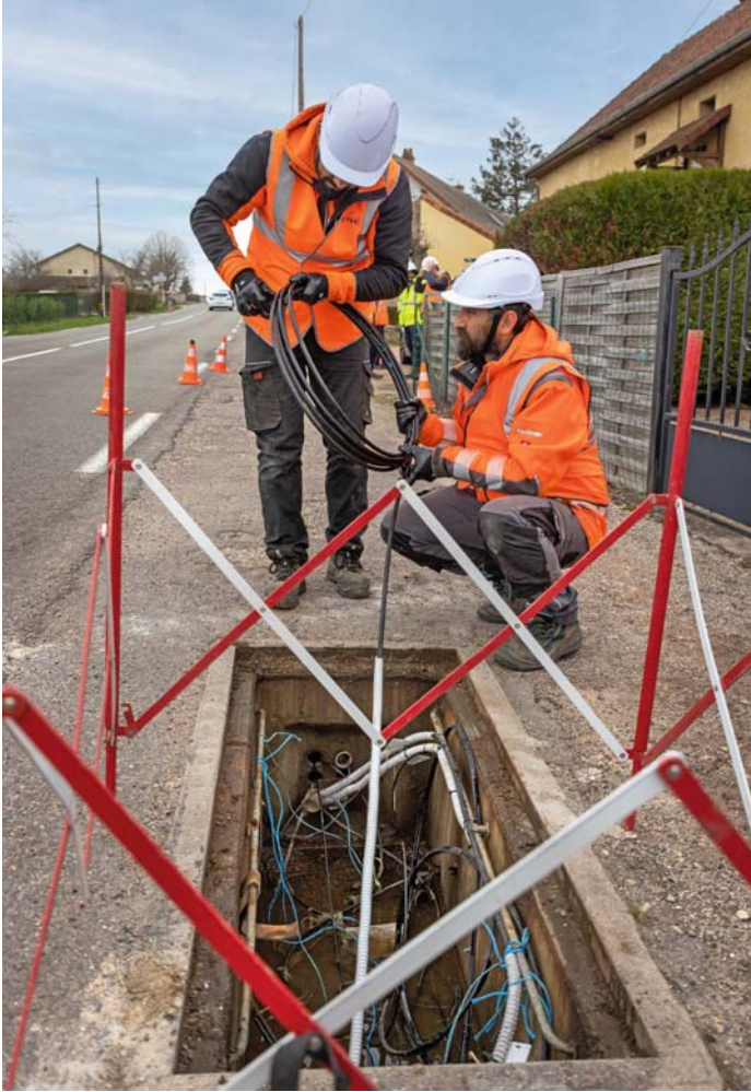
← Fiber optic cable is pulled by hand over several kilometers.
