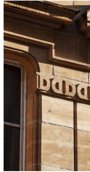
↑ The rehabilitation of a building calls for stonecutters, roofers, carpenters, wrought-iron craftsmen, and other skilled workers.
