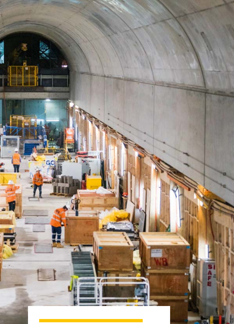
← Finishing works are underway at State Library Station.
