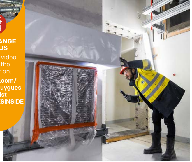
↗ Clément Pfund, an Equans project team member, checks the draught proofing.
