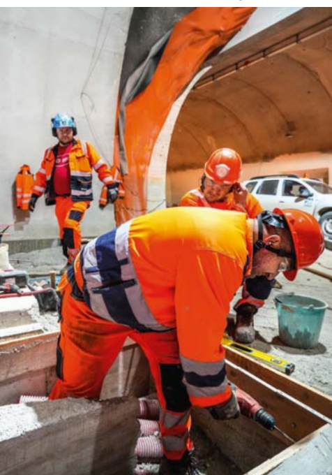
↓ A team working on the roadway.
