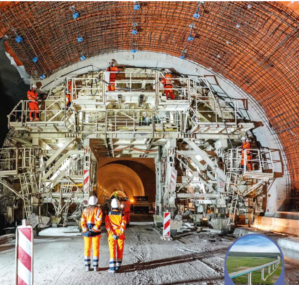
← Formworks used in shotcreting inside the tunnel.
