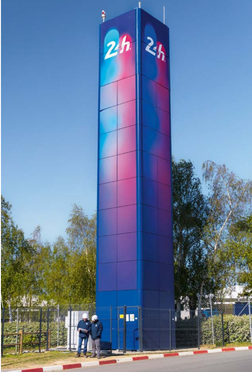
↑ A Bouygues Telecom antenna tower at the center of the circuit displaying the colors of the 24 Hours of Le Mans.
