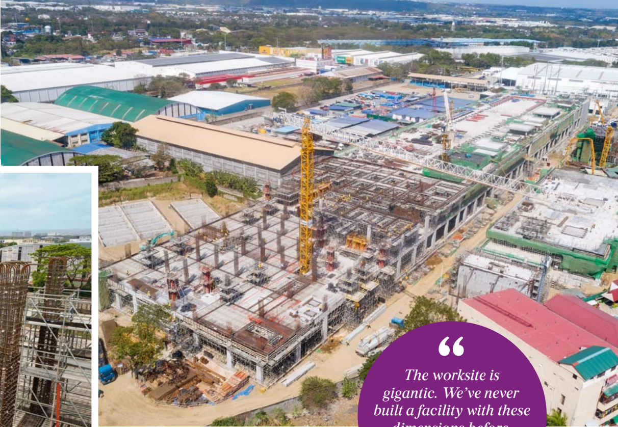
→ Construction of the main building, which will be 325 meters long and 55 meters wide.
